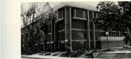
The Clement C. Maxwell Library, opened in 1971, is the College's newest building. The building has the capacity to house 425,000 volumes within its large and impressive four stories, and can accommodate 2,500 students. Among its features are a host of sophisticated research facilities, including an extensive collection of microfilm and microfiche holdings, a dial-access carrel system which allows students to view and listen to specially prepared films and tapes for selfpaced learning, and a special collections department of rare books.
